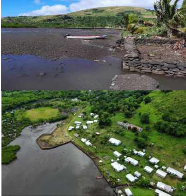
Figure 42: Project site at Nayavutoka Village
