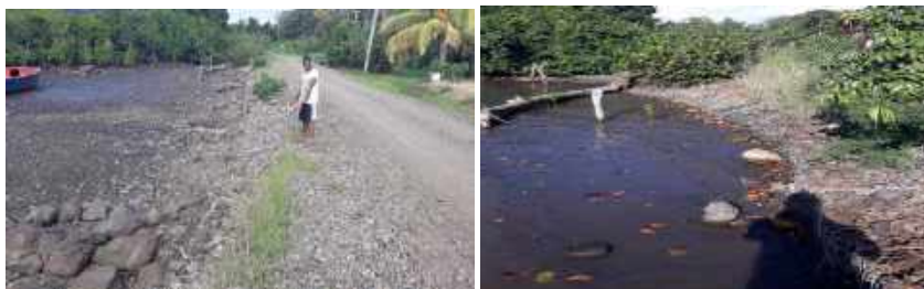
Figure 28: Project site at Namama Village
